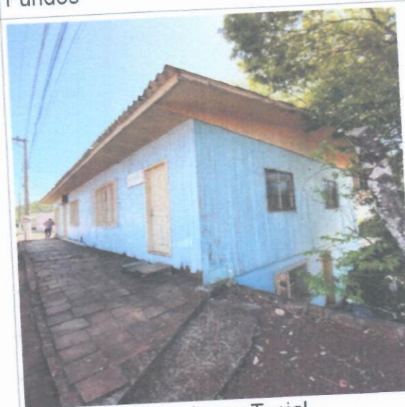
Lateral Rua Domingos Tonial
